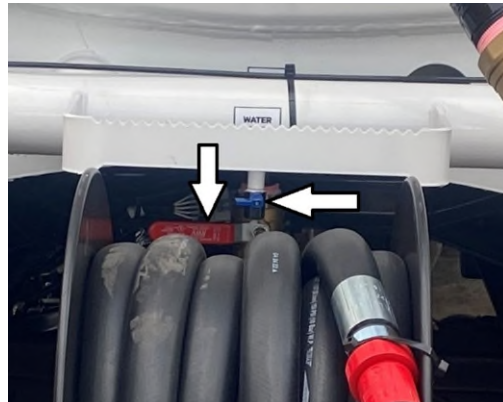
Rear Spray Bar & Tank Drain Valves
